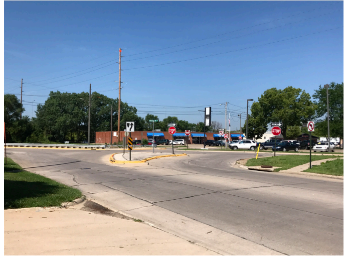
Figure 20: E Avenue NE & Oakland Road NE
